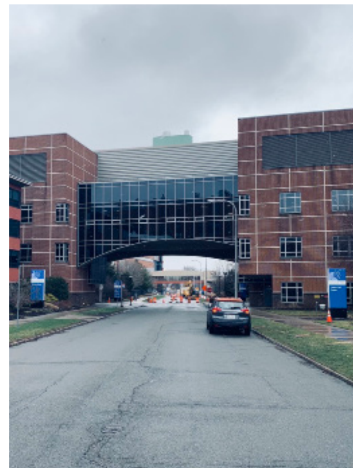
After a comprehensive visualization and sign management process, the final sign installation matches the digital visual simulation exactly.
