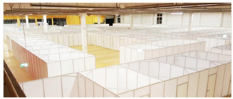
COVID-19 Modular Emergency Medical Rooms. Our partitioning wall system is modular and simple, made from panels and upright beam extrusions. Sizes to accommodate 2-3 beds available. Available with opaque sides. Graphic packages are available with ID SignSystem's patented Patient Communication Boards as well as Wayfinding and Room Identification Systems.
