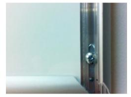
1. Open snap frame and mark wall with pencil through pre-drilled holes.
