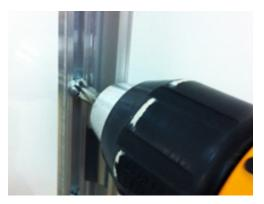
3. Be sure screw is secure and down completely. This will ensure that the frame will close upon completion.
