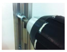
2. Use round head 2" screws. A plastic wall anchor is recommended.
